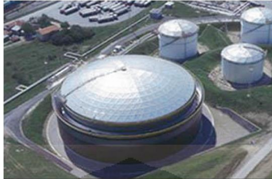
Gambar 5. Dome Roof Tank
